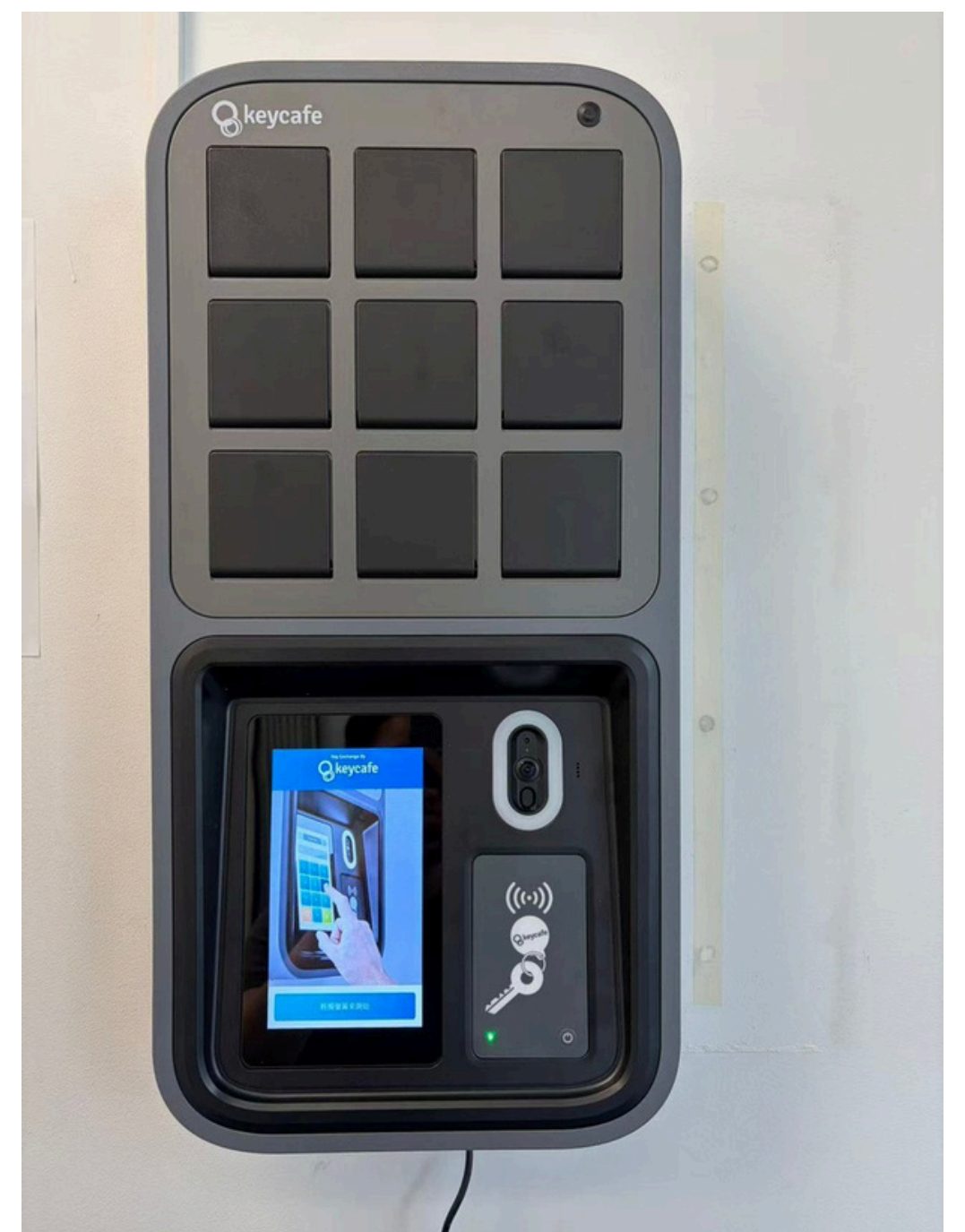
2. Find the key-box (Against the wall on your right-hand side)
